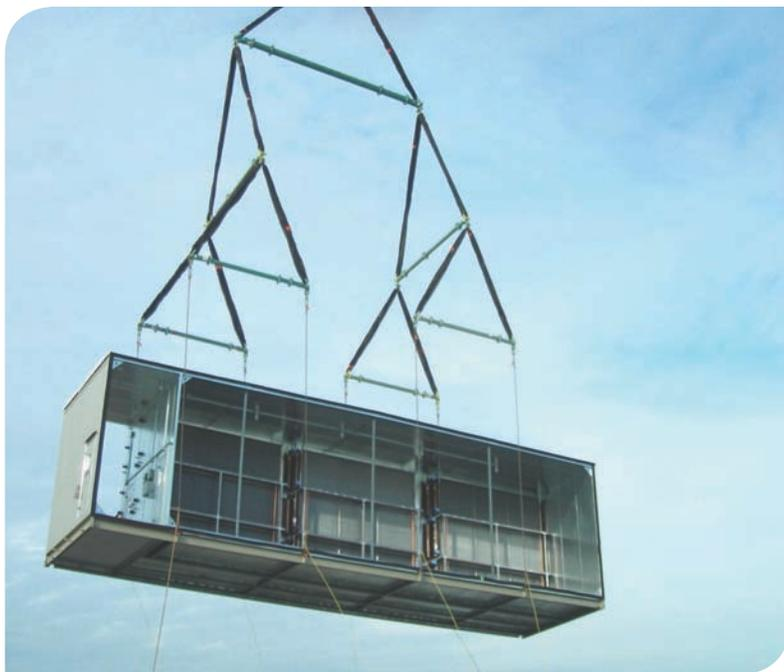
*Many Trane custom units are shipped completely assembled, ready to rig into position with one single-point power connection.*
